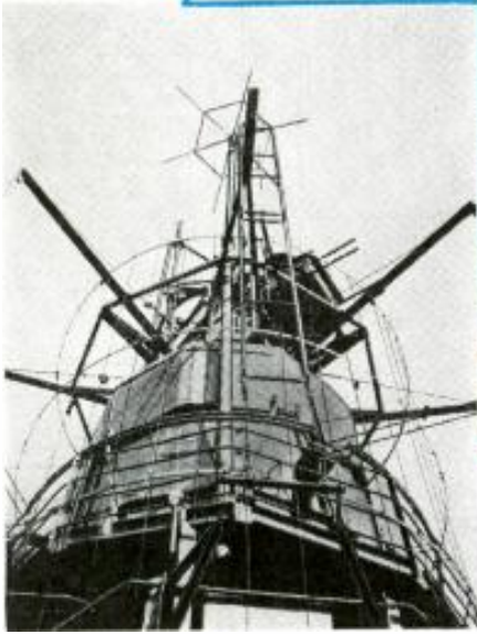
The Eiffel Tower bristles with TV antennas. Ladder enables workmen to reach the elements.
