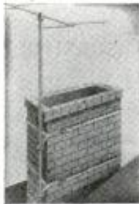
Fig. 12 (above)—South River antenna chimney mount has metal straps.
